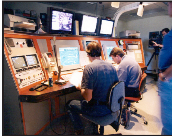
Tests are monitored from the Command, Control and Data Acquisition System building.
